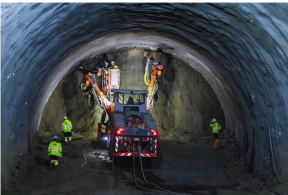
Faster and more efficient: LEAN means better cooperation © PORR
