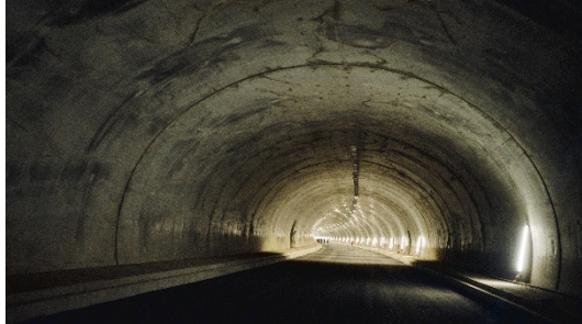
Civil Engineering Tunnel TS 26
