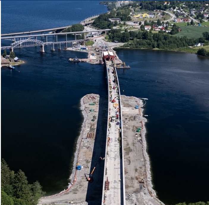
Infrastructure Minnevika Bridge, NO
