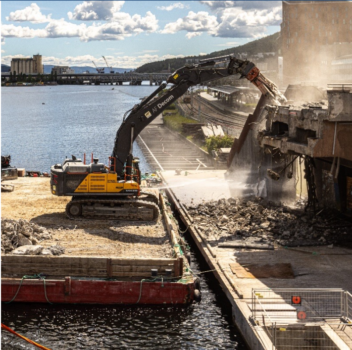
Demolition Drammen Bridge, NO 2022
