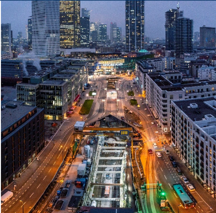
Tunnelling U5 Tramline Frankfurt, DE
