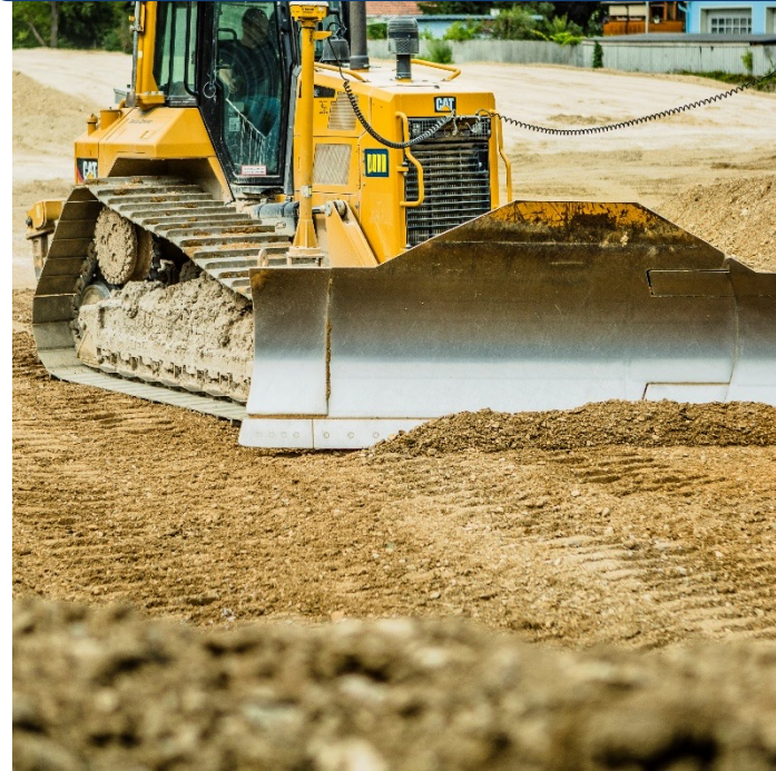
Earthworks HWRHB Fahrafeld, AT 2020-2023
