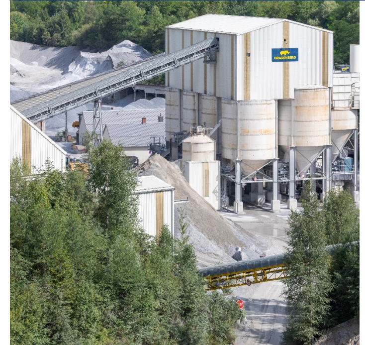
Stone Quarry Gradenberg, AT wholly owned PORR subsidiary since 2005
