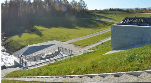
Special Projects Flood retention basin Roztoki
