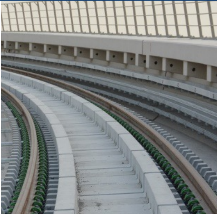
Slab Track Metro Doha Greenline, QAT
