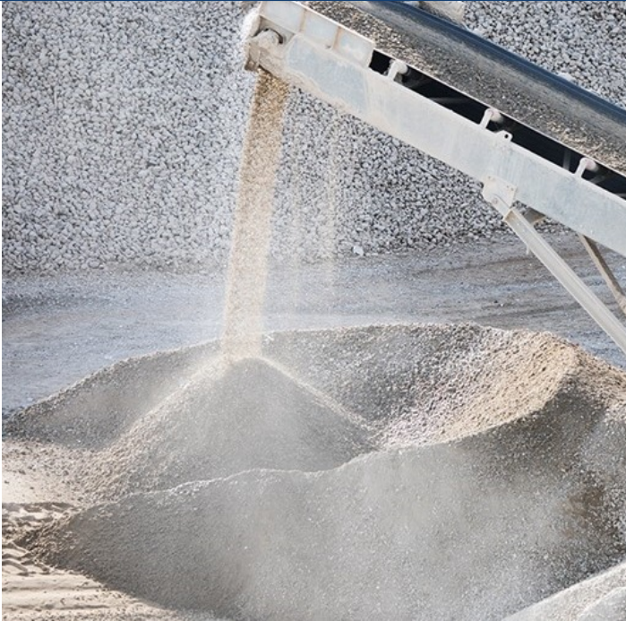
Gravel Washing Plant Himberg, AT in operation since 2010
