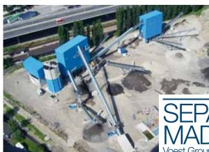
In the city of Linz PORR operates a wet screening plant and concrete mix plant as part of a consortium. The wet screening plant processes excavated material on the compound of voestalpine Stahl GmbH. It also produces certified products for the construction industry and aggregates for concrete mix plants.
