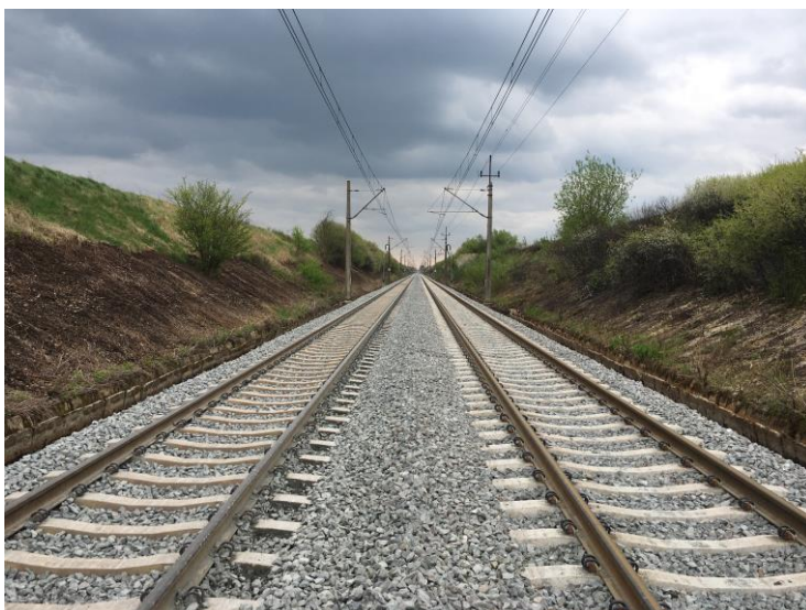
Caption: PORR demonstrates infrastructure expertise in Romania (Copyright: © PORR)
