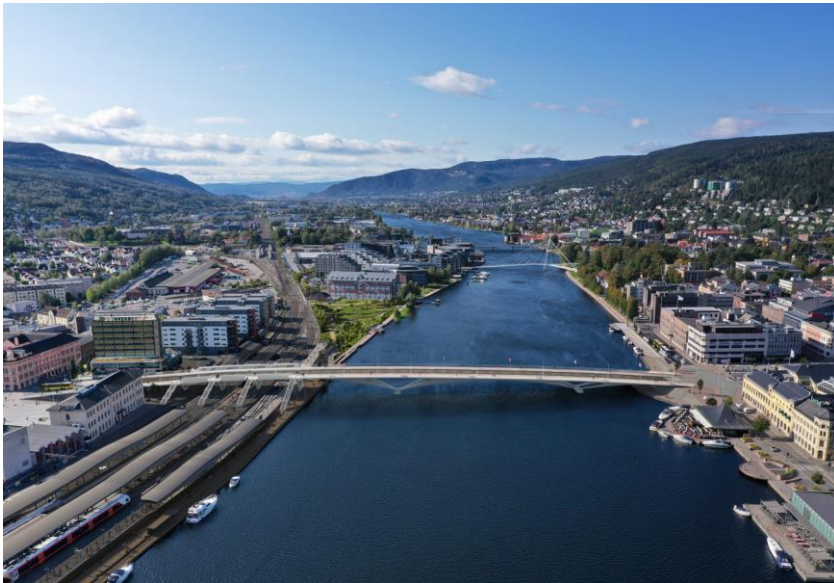
New city bridge in Drammen © Degree of Freedom, SAHAA, Knight Architects, Norconsult og Asplan Viak
