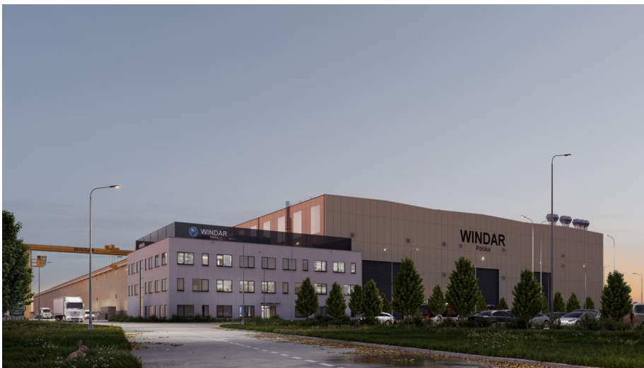
Planning and construction supervision was carried out by Industria Project Sp. z o.o. from Gdańsk, a planning company specialising in industrial construction © Industria Project
