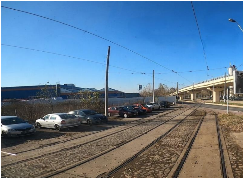
The rail infrastructure is showing its age - PORR will give it a complete overhaul © PORR
