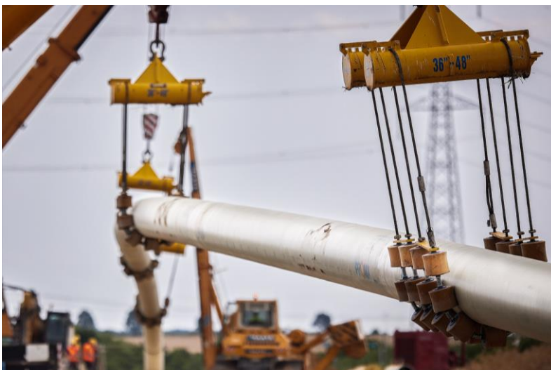
The high-pressure natural gas pipeline has a diameter of 1 m © PORR
