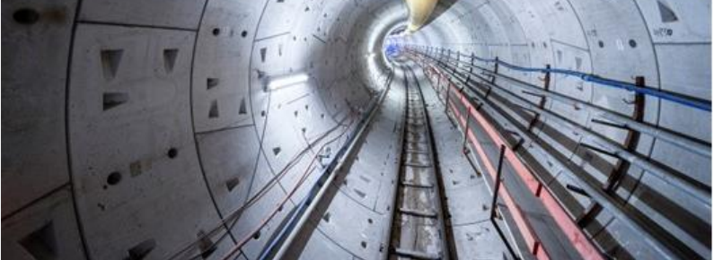
RAIL INFRASTRUCTURE KAT3- Koralmtunnel
