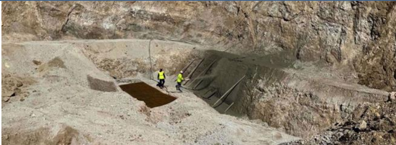
STORAGE OF ELECTRICITY PSKW Ebensee
